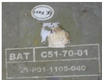
Figure 51.66. Battery box front plate with “QC pass” sticker
