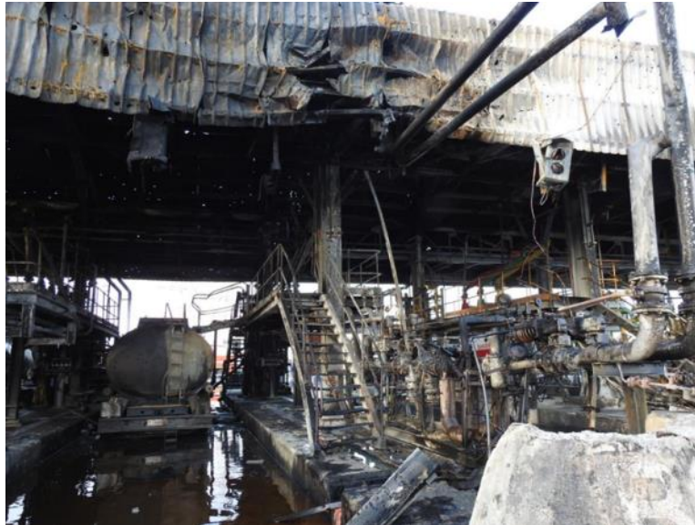
Figure I Abu Dhabi National Oil Company facility attacked on 17 January 2022
